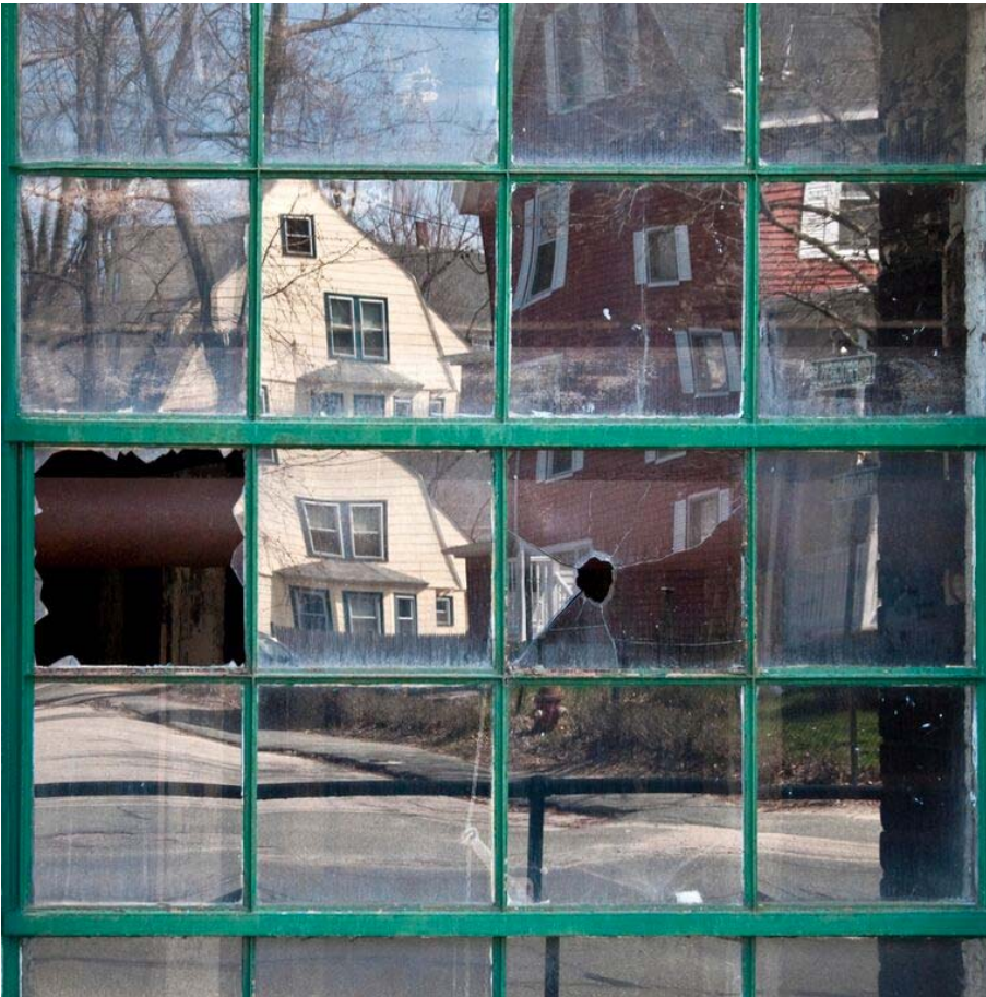
Progress Road archival photograph on aluminum 24x24" $625
